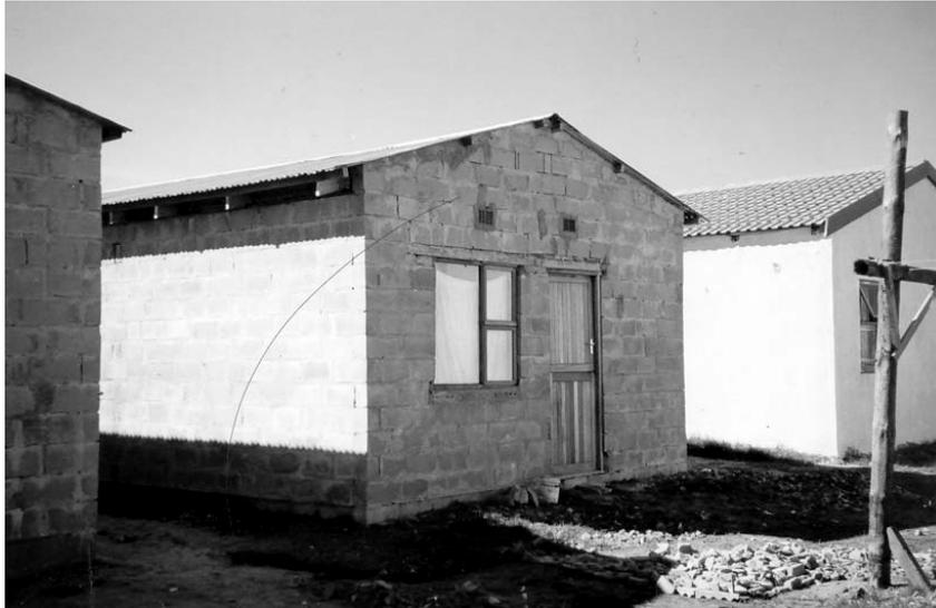
*Fig. 1: Noma's house with some of the problems visible, area above the wall and below the roof not filled in, no ridge piece, bad workmanship above door and window.*
